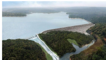
WEATHER July 24, 2011 Hundreds of People Missing after Dam Collapses in Laos
